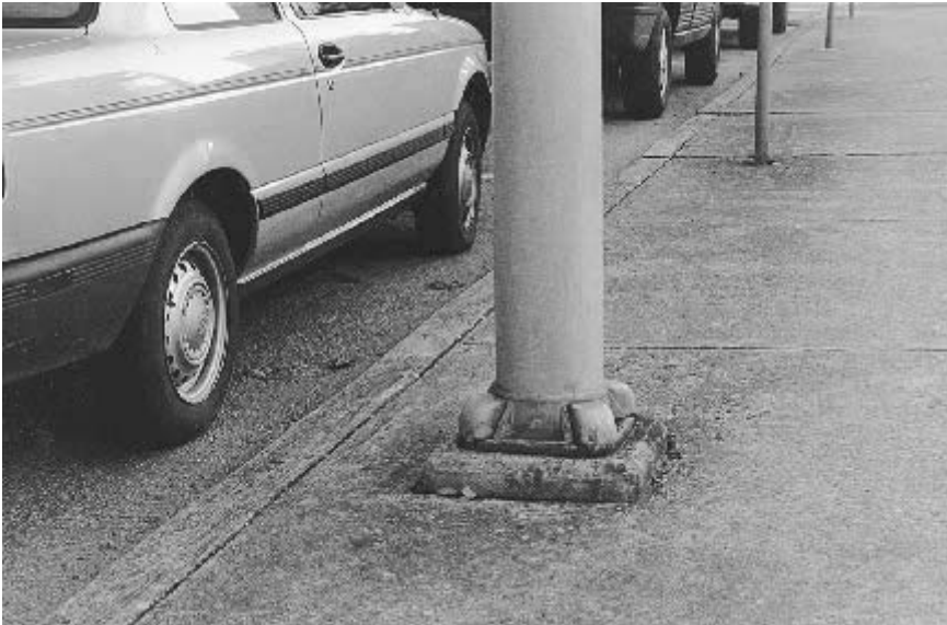
FIGURE 7.89 Flange-type steel base.
