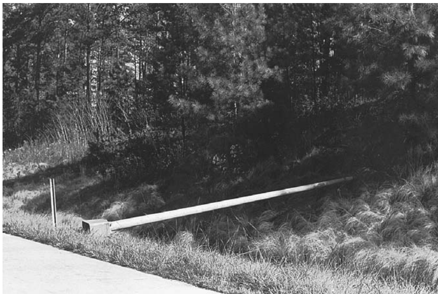
FIGURE 7.95 Failure of luminaire support without impact.
