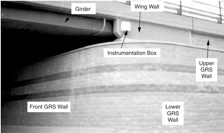
FIGURE 8.64 View of southeast side of the Founders/Meadows bridge abutment. (From Research Report, Colorado Department of Transportation, Denver, Colo., with permission)
