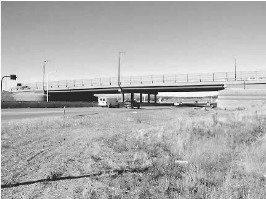
FIGURE 8.63 View of Founders/Meadows Bridge near Denver, Colorado. (From Research Report, Colorado Department of Transportation, Denver, Colo., with permission)
