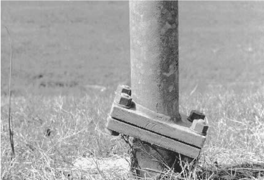
FIGURE 7.27 Installation of unidirectional slip base.
