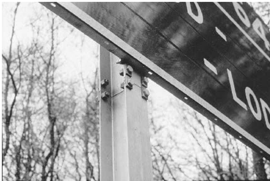
FIGURE 7.40 Commercially available hinge plates by Transpo Industries.
