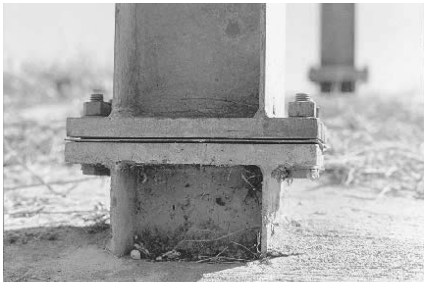
FIGURE 7.34 Installation of horizontal slip base.
