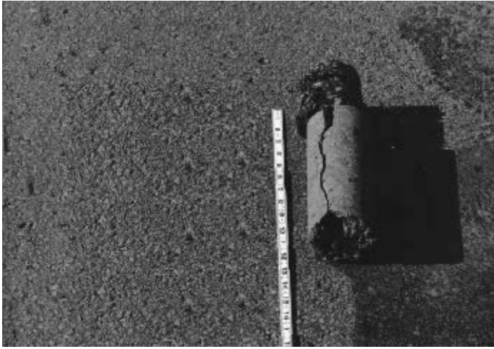
FIGURE 3.41 Pavement core taken at transverse joint in composite pavement.
