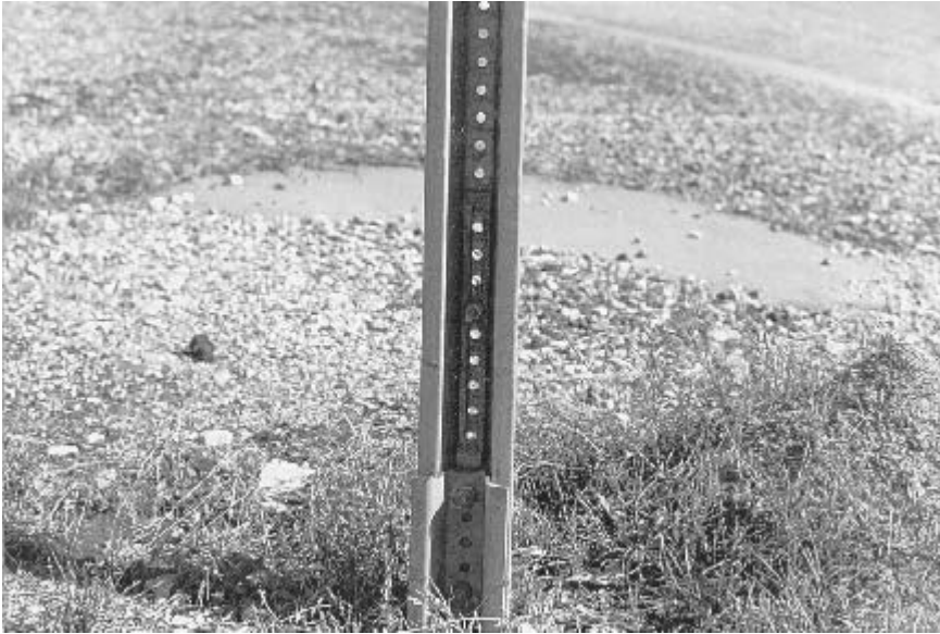
FIGURE 7.7 Example of breakaway single sign support.
