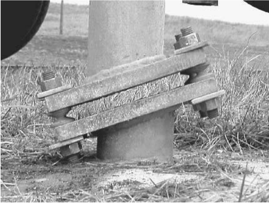
FIGURE 7.30 Frangible-coupling sign support.
