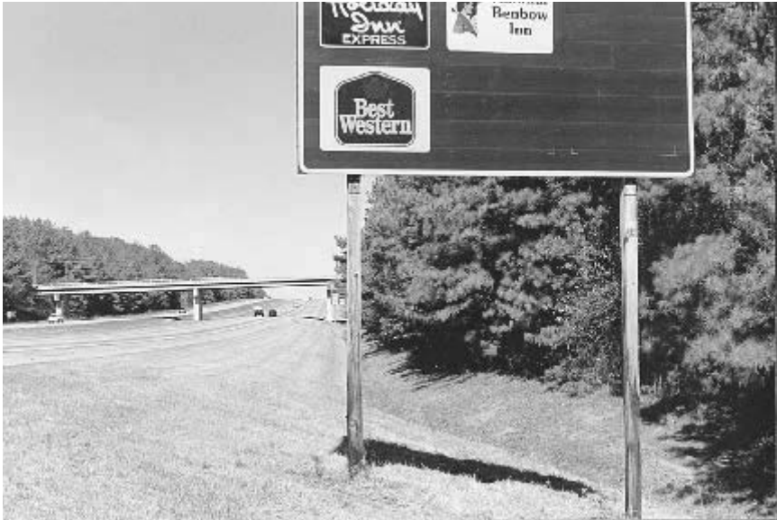
FIGURE 7.61 Multiple-mount frangible wood post design.
