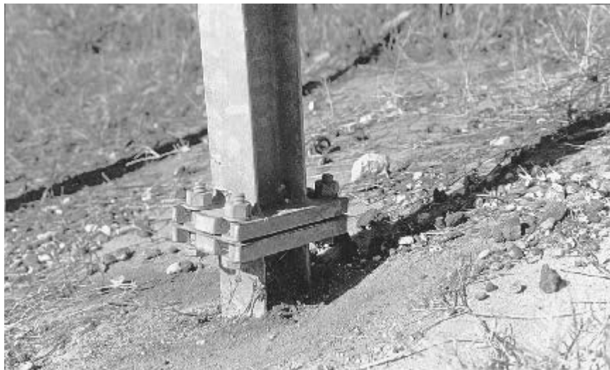
FIGURE 7.8 Example of mechanical release support type.
