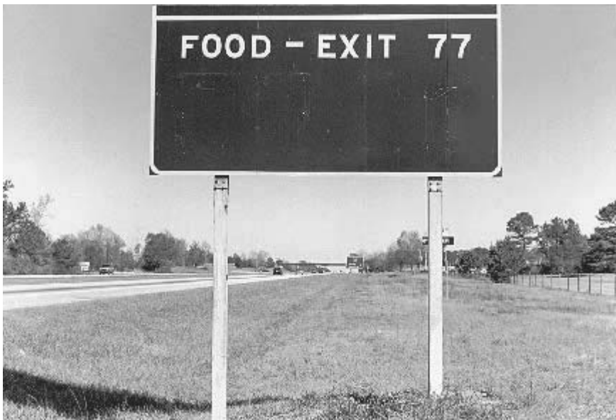
FIGURE 7.31 Multiple-mount sign support.
