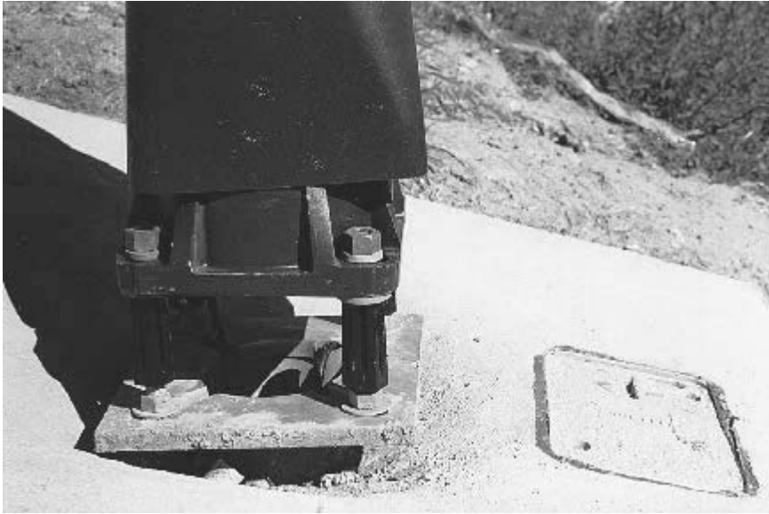
FIGURE 7.90 Frangible-coupling luminaire support.
