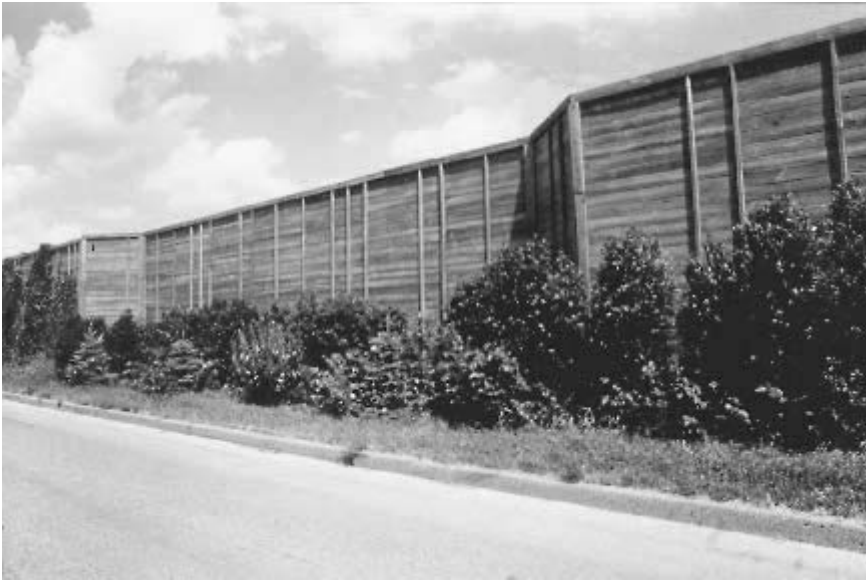
FIGURE 9.4 Timber noise wall with buttress-type alignment.
