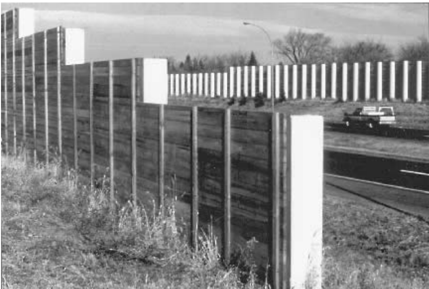
FIGURE 9.5 Timber noise wall with concrete posts showing effect of contrasting hues.
